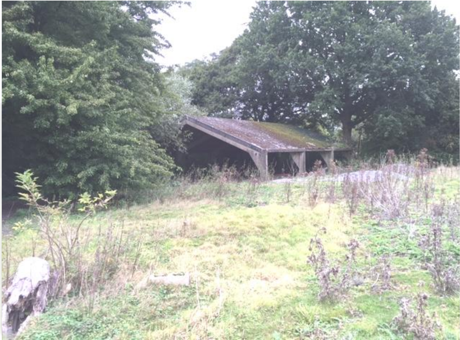
Photo 10 : View of open sided barn facing north east
